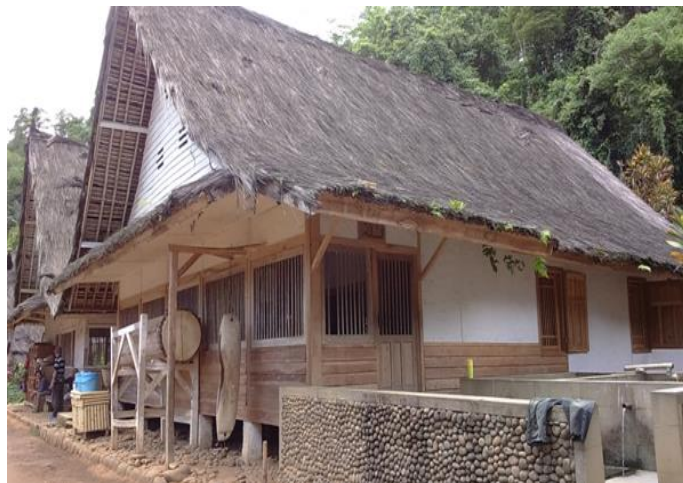
Figure 4: Roofs for a Mosque made from sugar palm fibres in Kampung Naga, Tasikmalaya, West Java
