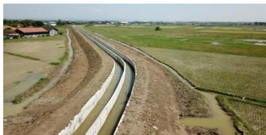
Gambar 3. Double U-Ditch Precast
